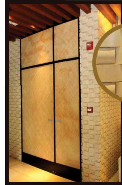
◀ Engineered Stone in brick profile gives accent to the blind door in wallpaper finish with solid teak wood door frame view.
