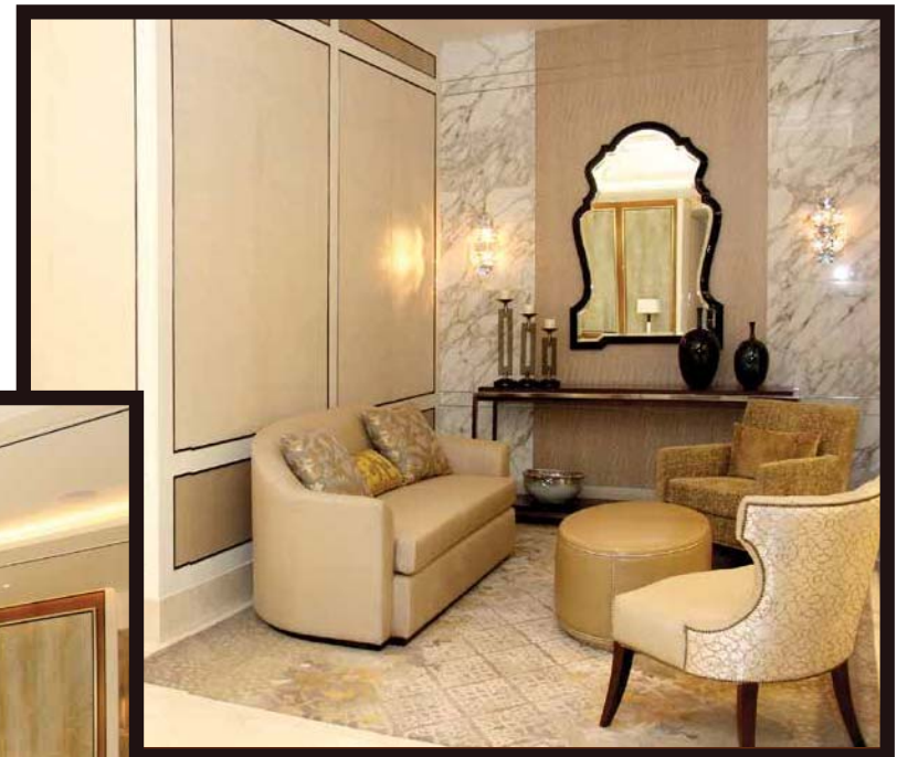
General wall in special veneer finish, matched with special wallpaper and terminated by a 5mm x 5mm blackened metal insert
